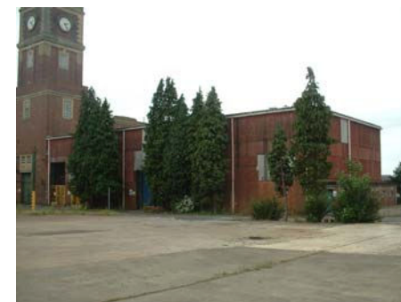
Fig. 3 Later extension to Boiler House
