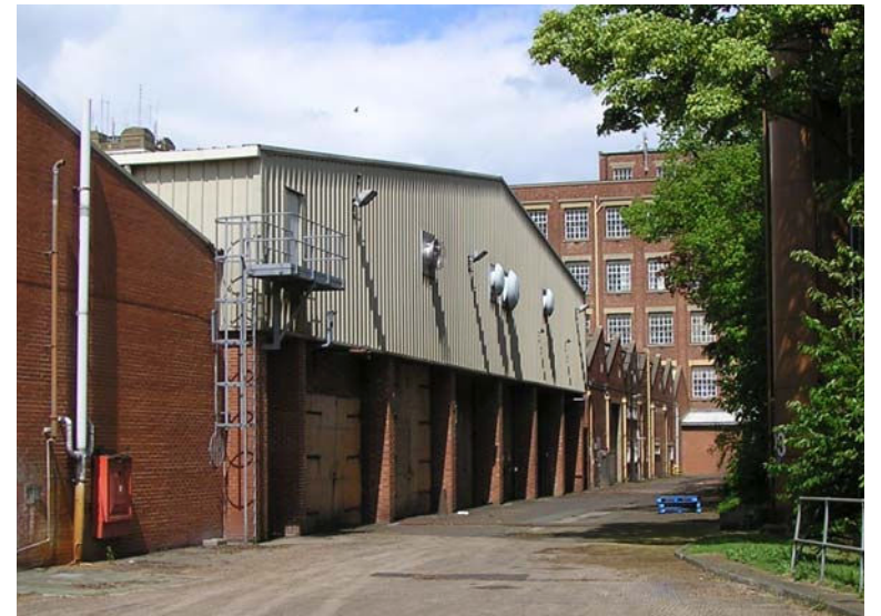
Fig. 45 View looking north-west within factory grounds
