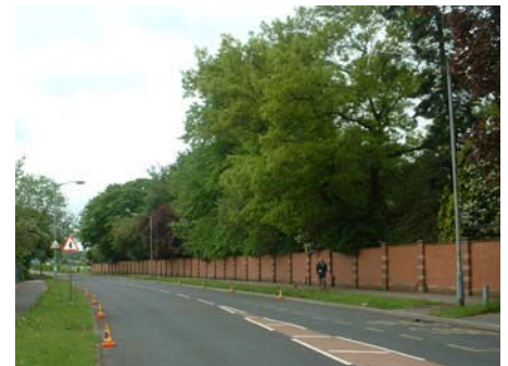
Fig. 6 Existing eastern boundary along Bishopthorpe Road
