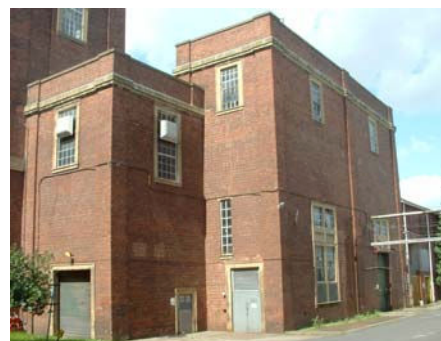
Fig. 53 Boiler and Transformer house
