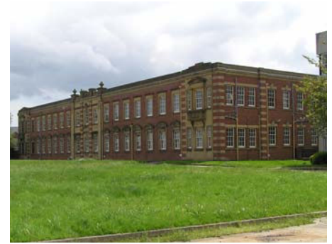
Fig. 4 Line of existing boundary along the northern elevation of Head Office
