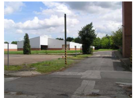
Fig. 5 Northern section of factory site
