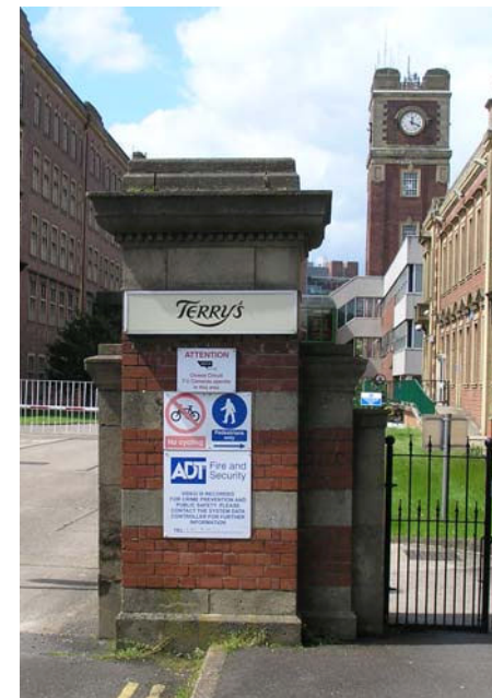
Fig. 58 Inappropriate signage at main entrance
