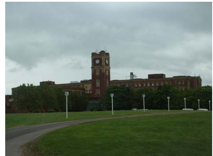
Fig. 40 View south-east across Park Pavilion Field
