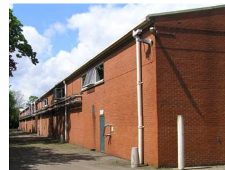
Fig. 56 Modern extension to north light shed
